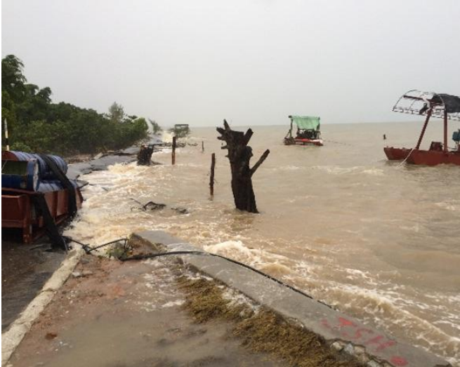
Coastal flooding caused by high tides and wave overtopping, inundating low-lying areas along the shoreline.
