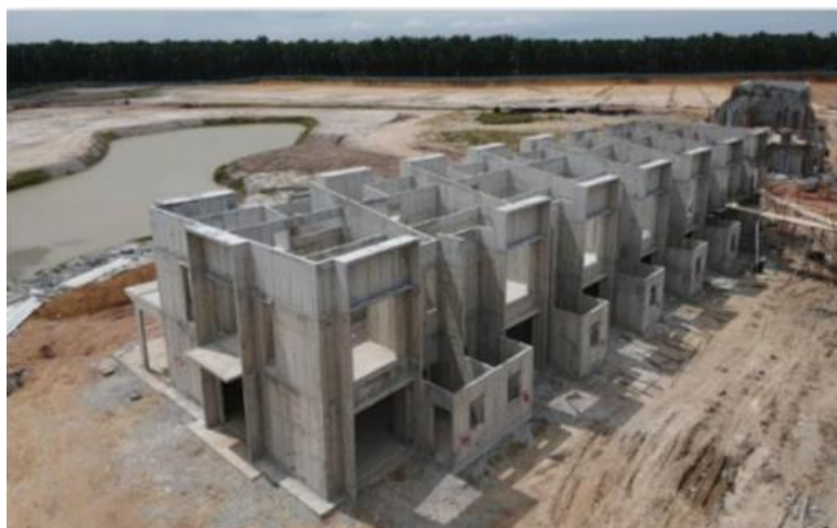
Aluminium formwork in Taman La Casa Lunas
