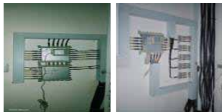
Satellite Master Antenna Television system
