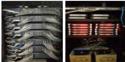
Satellite Master Antenna Television system
