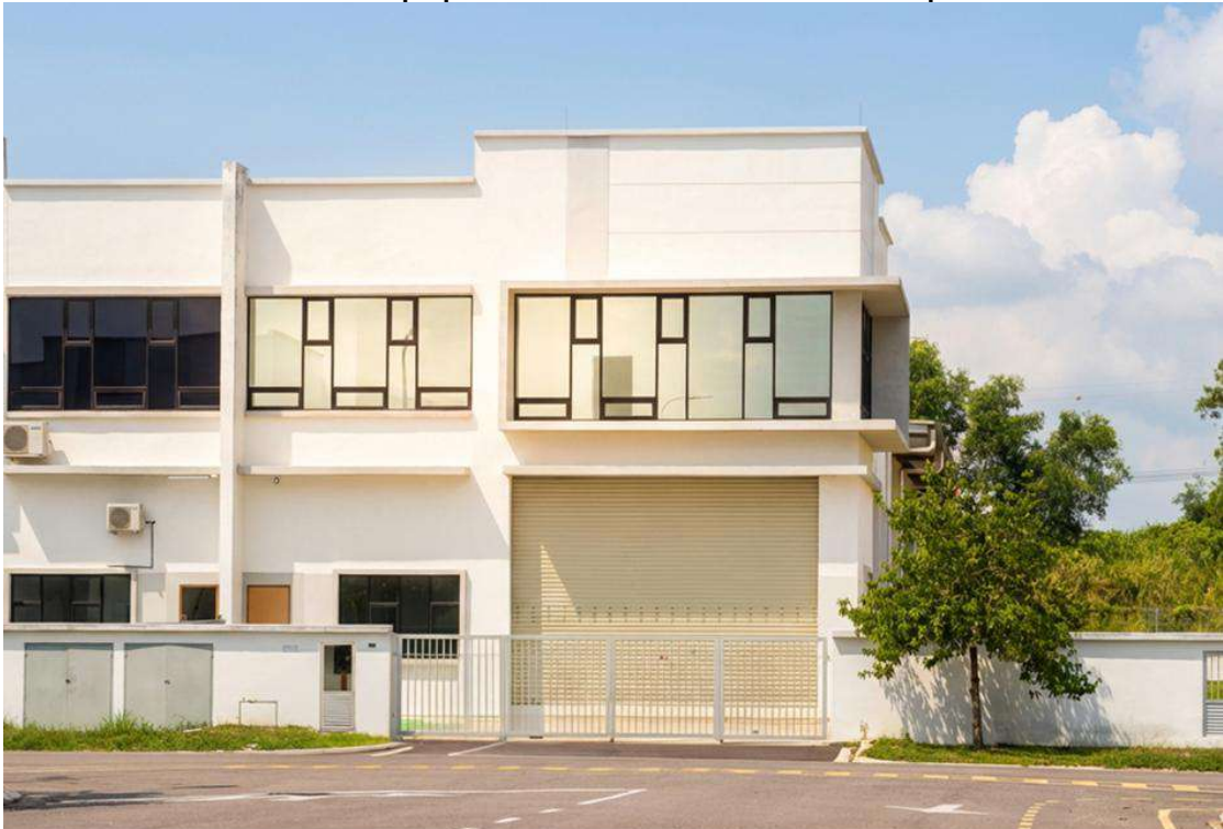
Industrial properties in Taman Bukit Perdana township
