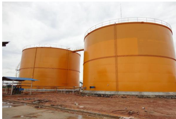
CPKO storage tanks
