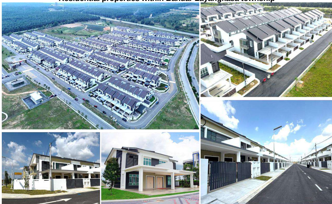
Residential properties within Bandar Layangkasa township
